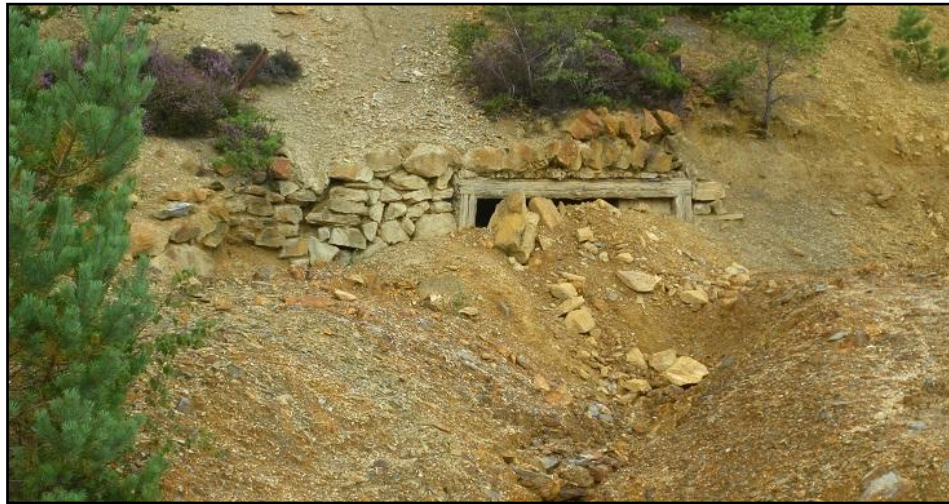
Timbered entrance to 850 Level adit partly hidden behind spoil. The channel in front was dug in recent years to accommodate a periodic discharge of water from the adit, a recent development possibly related to blocking of the normal drainage routes within the mine.
