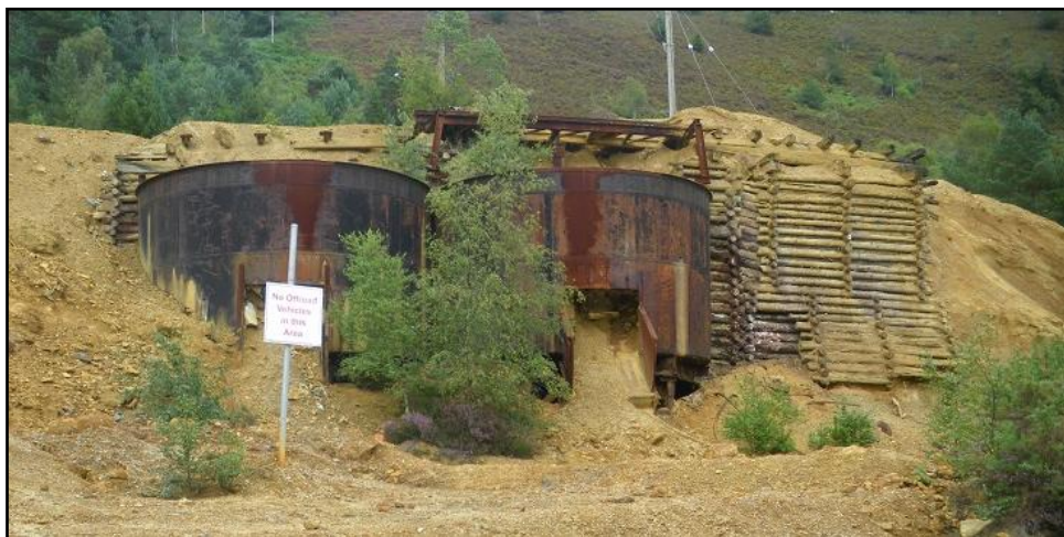
Ore bins installed in the late 1950s to hold ore trucked from the 850 adit and destined for the mill in West Avoca. One flatrod tunnel is located just to the right behind the bushes.
