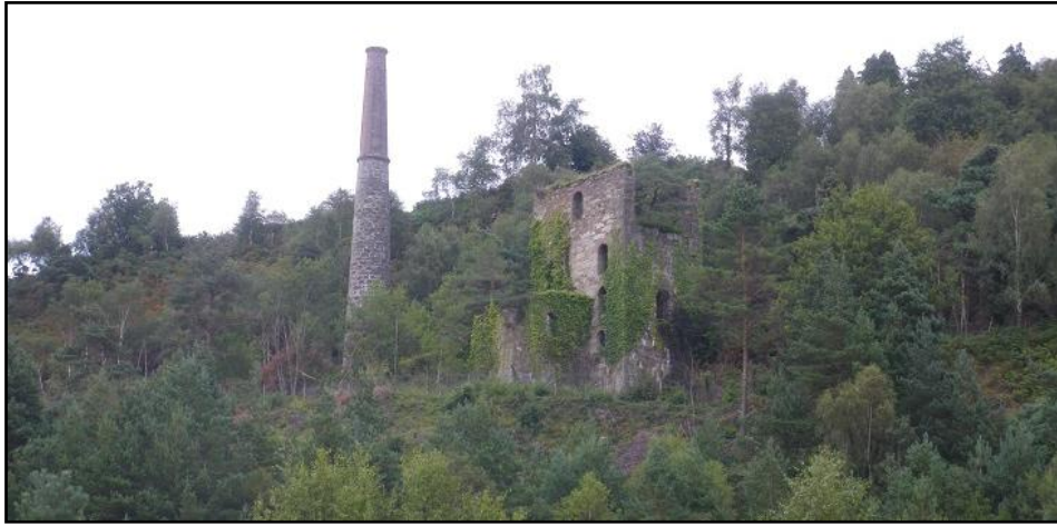
Williams Engine House, Tigroney West, viewed from southwest.
